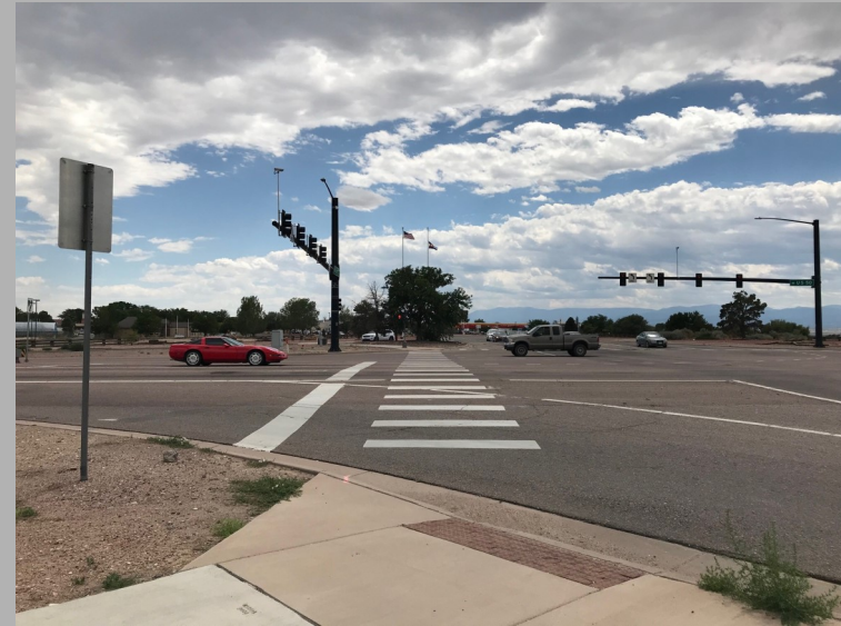
Highway 50 & McCulloch Blvd have crosswalks but due to width of both streets exposes pedestrians and bicyclists for a greater length of time when crossing.
