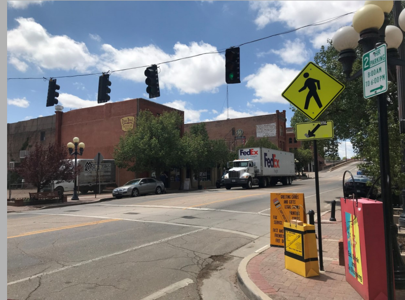
Mid-block crossing with a pedestrian accessible signal.
