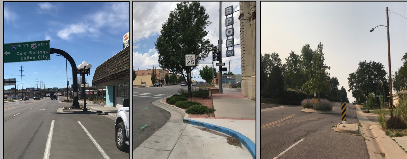
Images above from left & middle are examples of bump-out. Image above right is an example of small bump-out with a cut through for drainage and bicycles.
