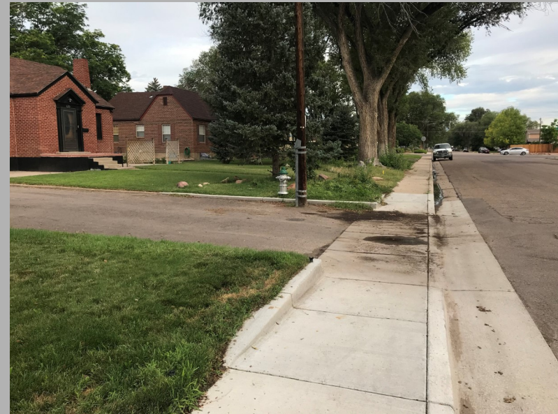
Curb cuts as shown above present access for people in wheel chairs or pushing a stroller.
