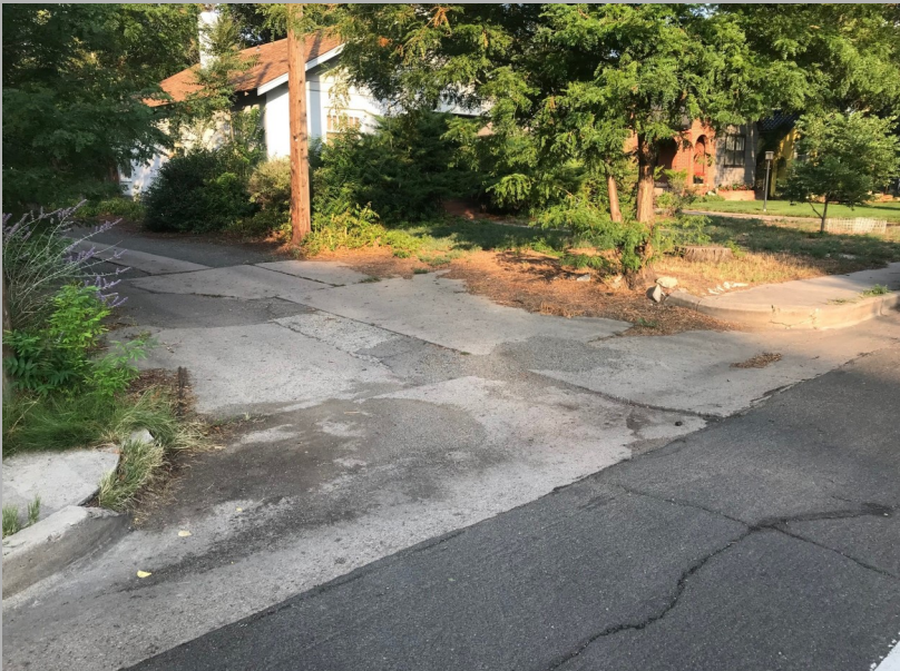
Lack of curb cuts make it difficult for users to cross between sidewalks.
