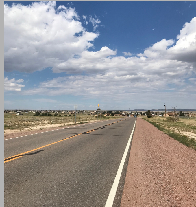
Image 3.2 Purcell Boulevard between Highway 50 and Platteville Blvd. Little to no shoulder for road cyclists.
