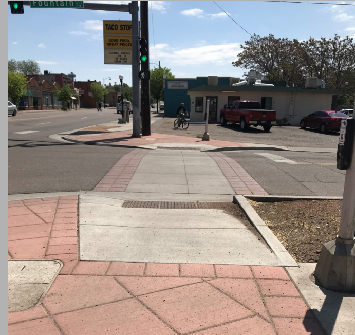
Image shows an intersection improvement with ADA curb ramps and accessible pedestrian signal.
