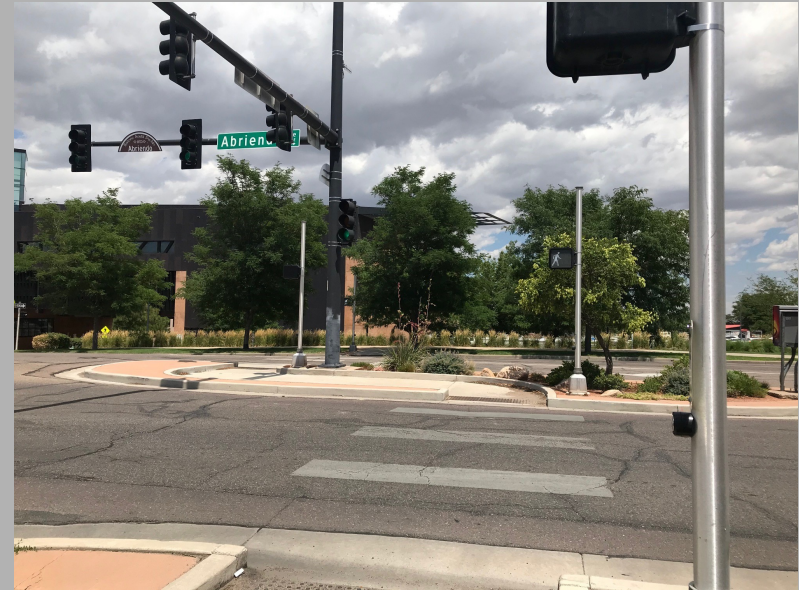
Pedestrian Island with pedestrian activated signal located at Abriendo Ave. and Broadway Ave.
