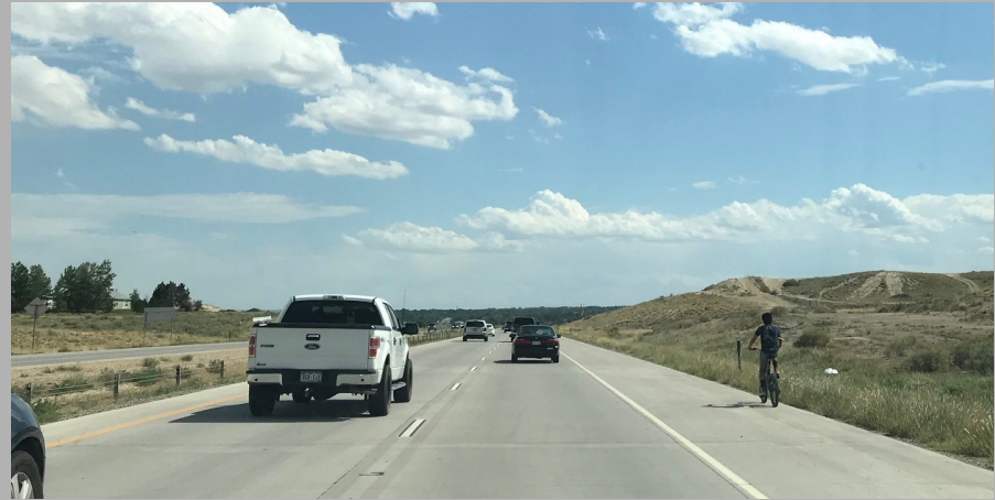
Image 3.1 Pueblo Boulevard between Highway 50 and 11th Street, both Northbound and Southbound lanes have 14' wide paved shoulders.
